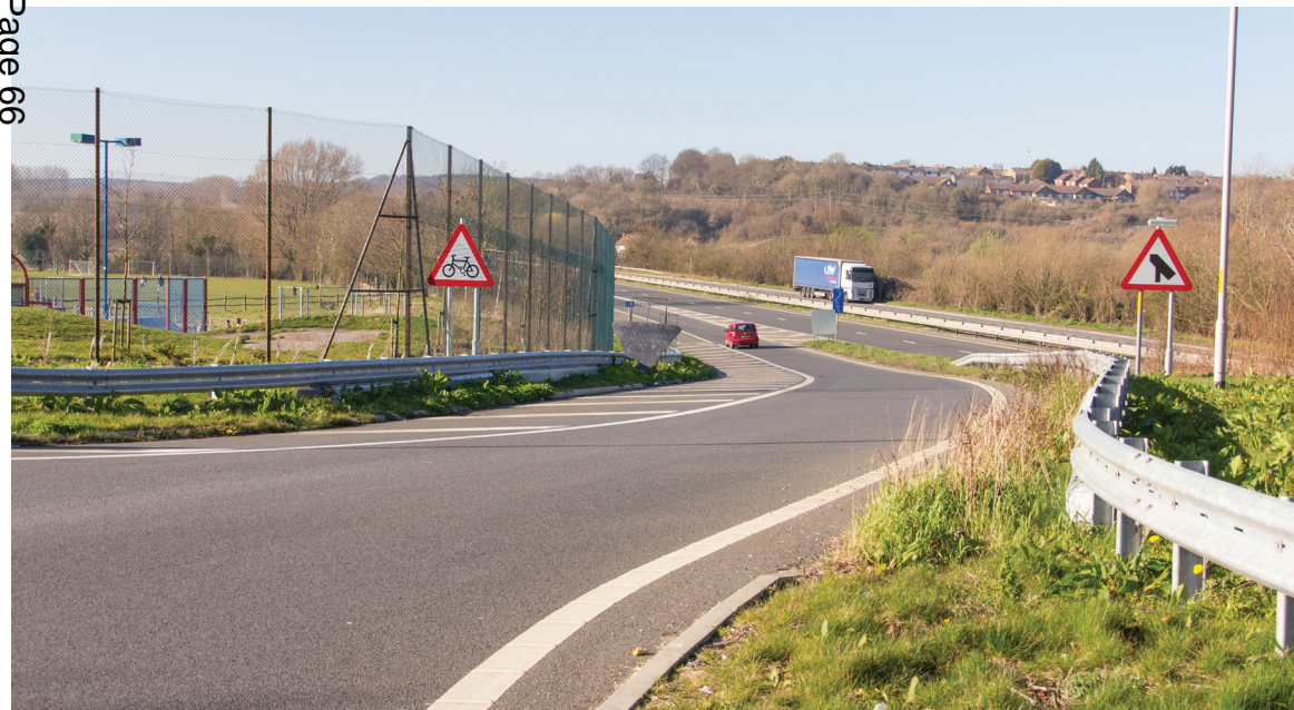
Figure 1.2 A2 London Bound On-Slip Road
